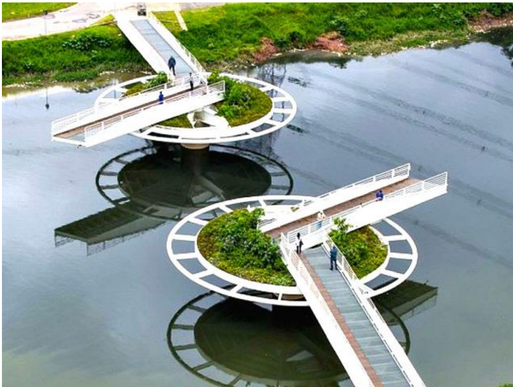
Figur 3-11 Friedrich Bayer Bridge [39]
